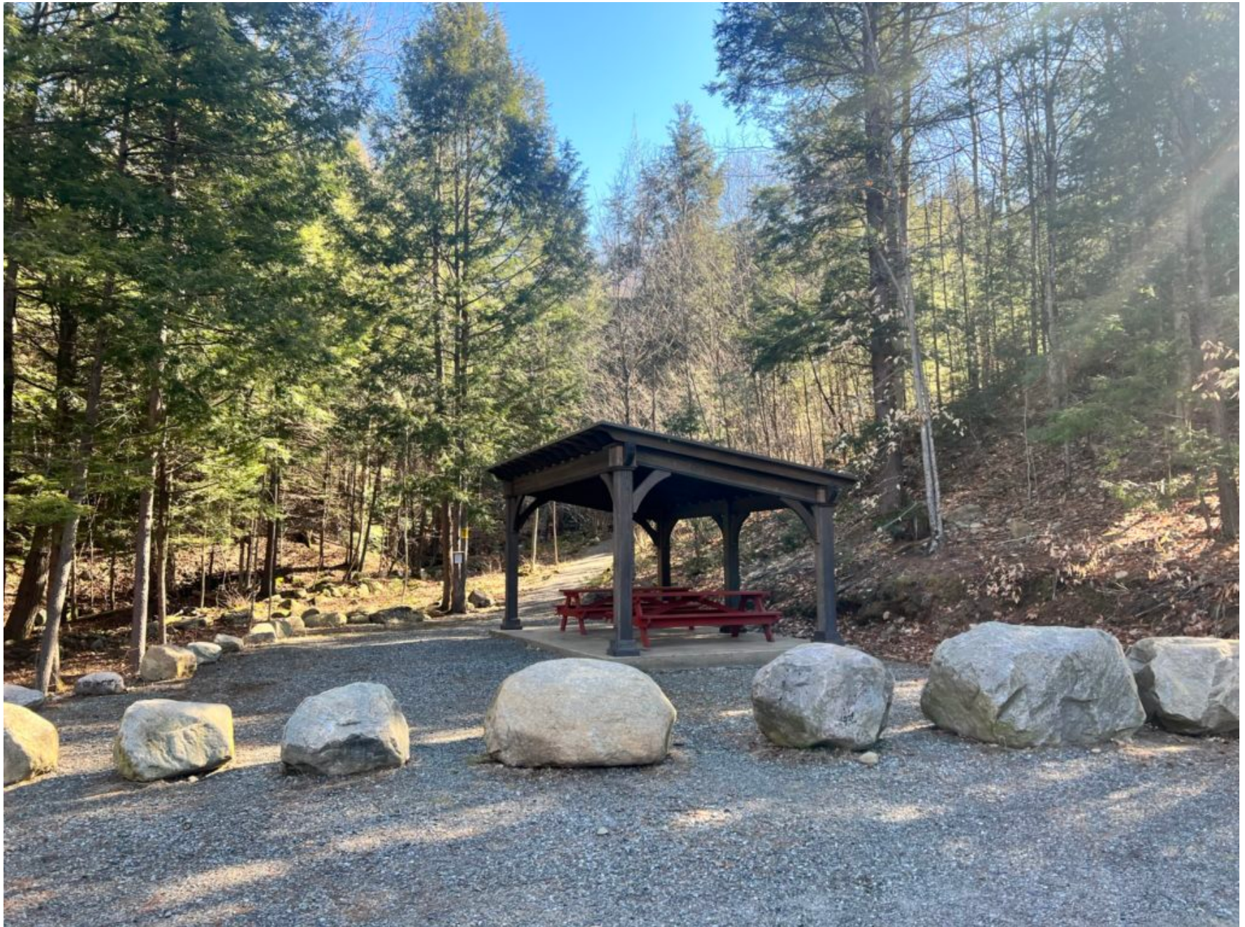
Potash Mountain Trailhead Shelter
